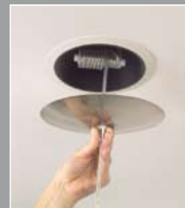
Slide up cover plate over recessed light.
